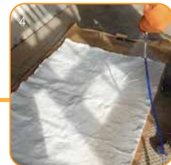
4. Spray on insulation fabric
