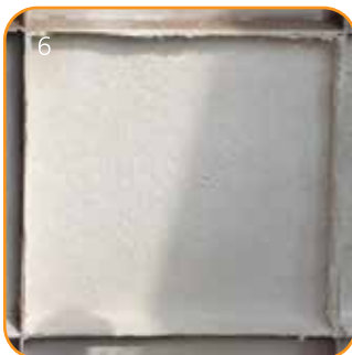
6. The second insulation spray (Final spray)
