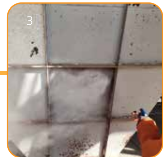
3. Primary insulation spraying on the surface
